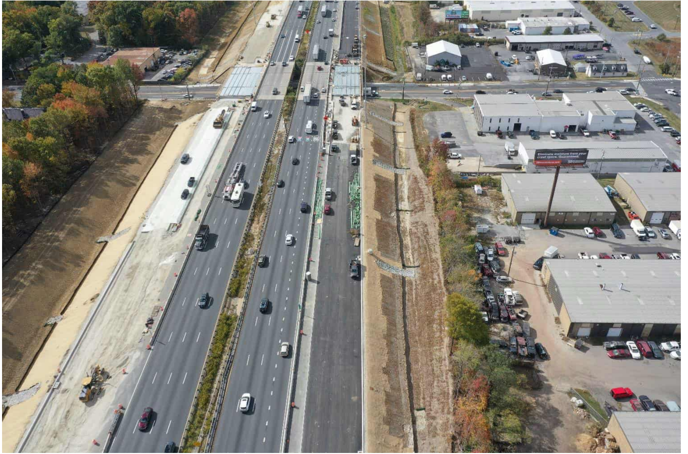
I-95 Widening Looking South
